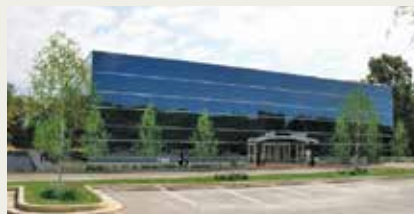
185 Admiral Cochrane Drive, Annapolis Maryland. 130,000 square feet of Class A office space.
