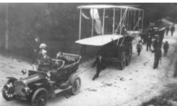
The Wright Flyer arrives at Ft Myer in 1908. The contract required that the airplane be quickly and easily assembled and taken apart and packed for transportation in Army wagons, taking no more than about one hour.
