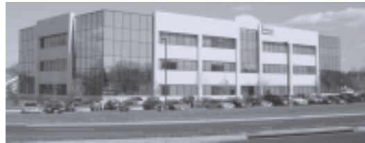
14150 Newbrook Drive – Completed in August 1999
