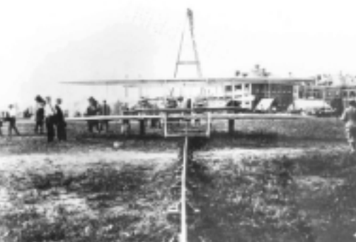
Launching the Wright Flyer was accomplished with a catapult (derrick shown in background). The plane was mounted on a 50 foot track with ropes attached to 1500 lbs of weights. The trigger for releasing the weight was pulled by the pilot. The Ft Myer Post Headquarters building can be seen in the background.
