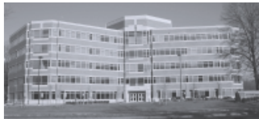
1775 Wieble Avenue – Completed in June 2001
